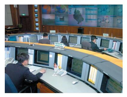
**Operations Centre** (WROC), operated by the Korean Water **Corporation (South** Korea) in Daegu, monitors water resources across the country, managing floods, water allocation and hydropower generation. Most of the hydrometric data network in South Korea is monitored remotely in real-time via a pervasive wireless network, supplemented by satellite-based communications (shown on screen).
