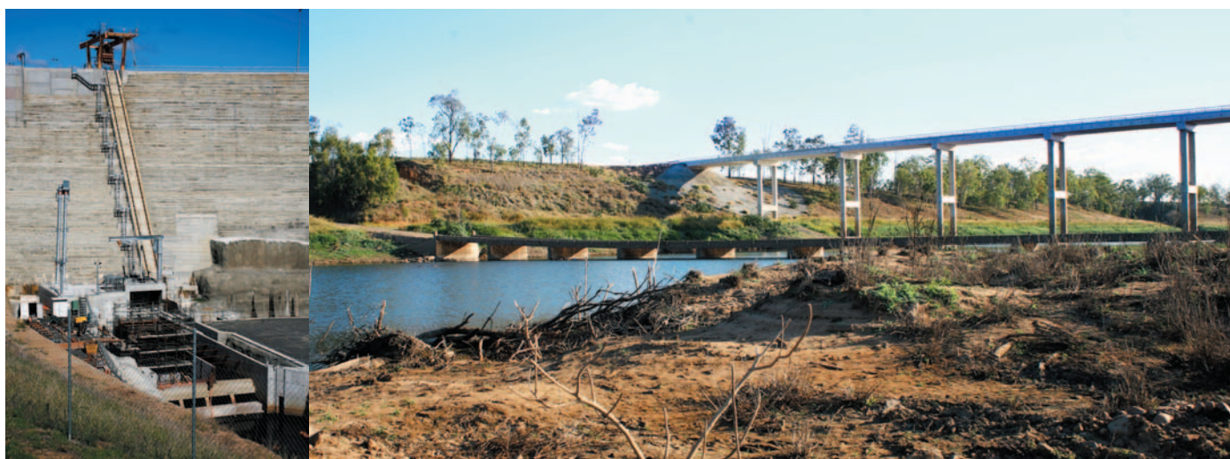
Left: A fish elevator and collection pool at Paradise Dam – there is considerable doubt as to its effectiveness. Right: Paradise Dam's backwaters at Mingo Crossing. The bridge suggests the full height of the dam, some 15 metres deeper than at present. Arkin Mackay, www.stoppress.com.au
