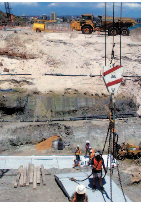
An excavation and construction site near Adelaide, showing darker sulfidic material (buried acid sulfate soil) at the foundation level. CSIRO Land and Water
