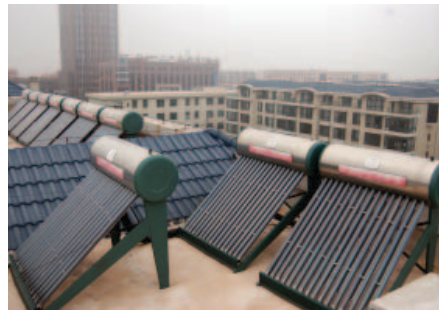
Solar water heaters populate the rooftops of most Rizhao buildings, thanks to local government subsidies for low-cost water heater manufacture. iStockphoto
