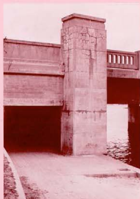
The result of alkali-aggregate reaction.
