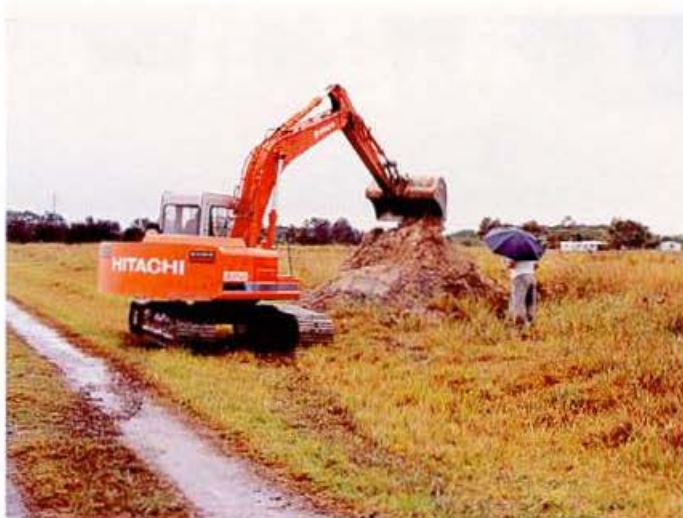
Excavating pits at Micalo Island so acid sulfate can be observed and sampled.
